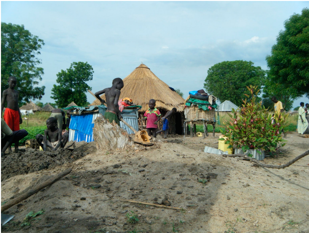
Figure 3. Digging up a termite mound for plaster.
